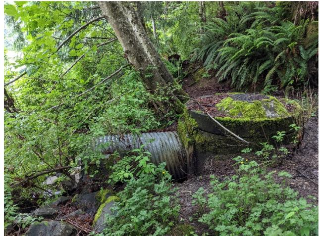
Photo 010: Stormwater outfall discharging to Davis Lagoon.
