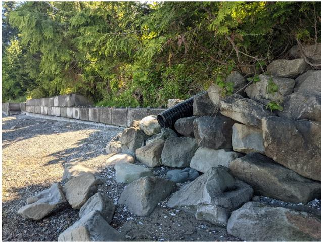
Photo 021: Stormwater outfall discharging onto beach SE of Gardner Road Beach Access.
