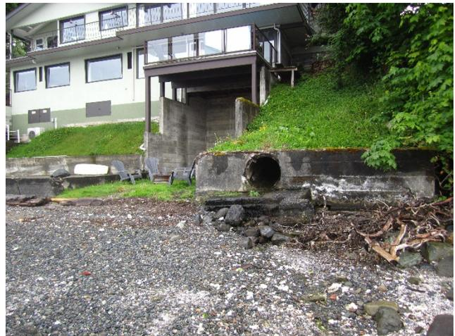
Photo 012: Stormwater outfall.
