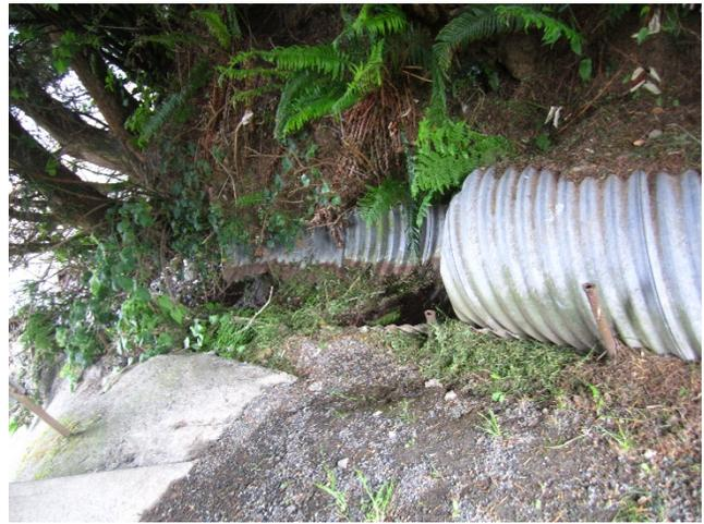
Photo 016: Stormwater outfall discharging to beach at Skinner Road Beach Access.
