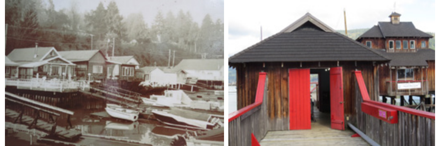
HISTORIC WOODEN STRUCTURES + RED TRIM
