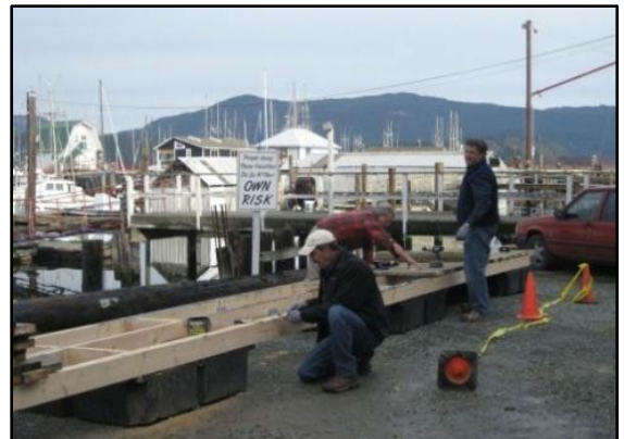
Photo: Dock construction for a Cowichan Bay marina (CVRD).
