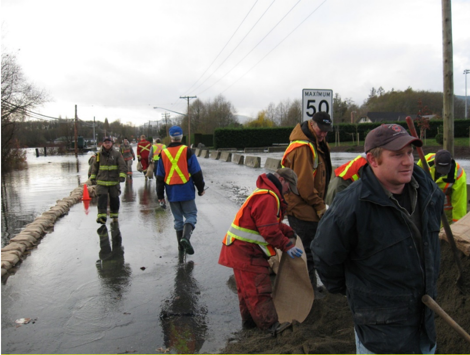
Photo 1: Construction of temporary no-post barrier on Lakes Road, Nov 20, 2009.
