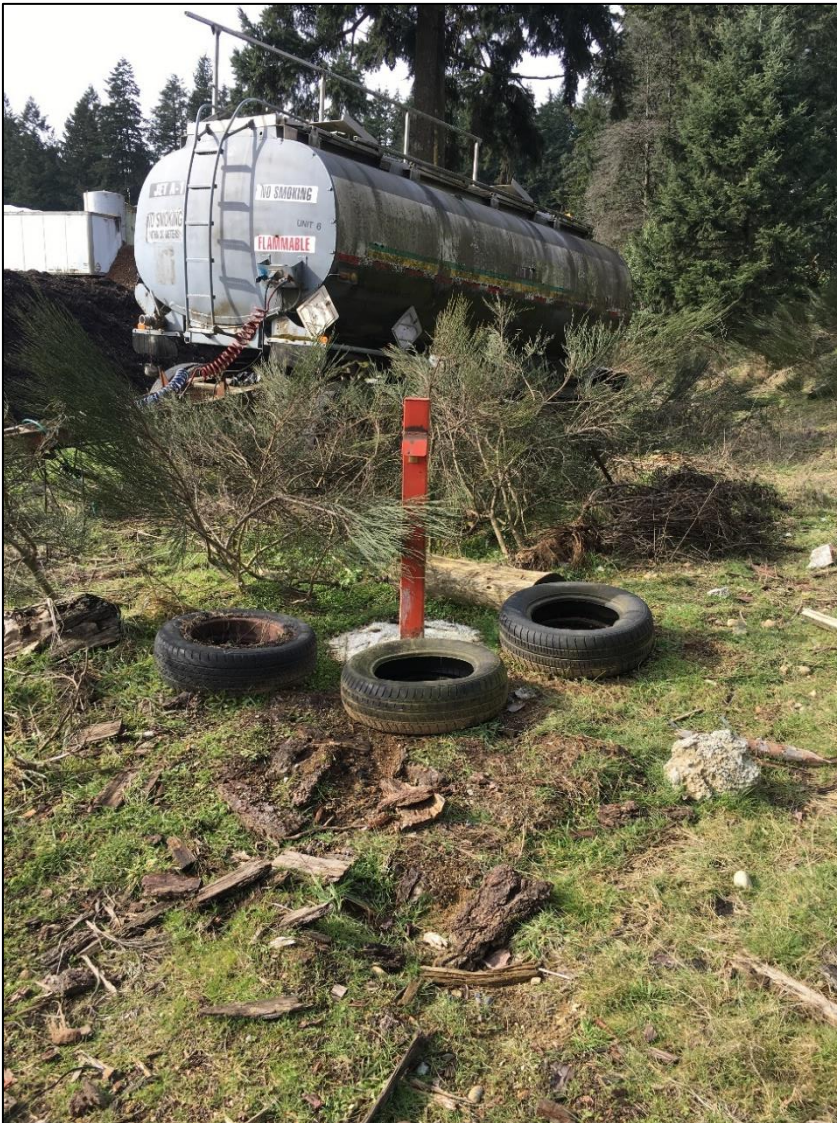
Photograph B3 (LEFT): Looking west at MW12-3.
