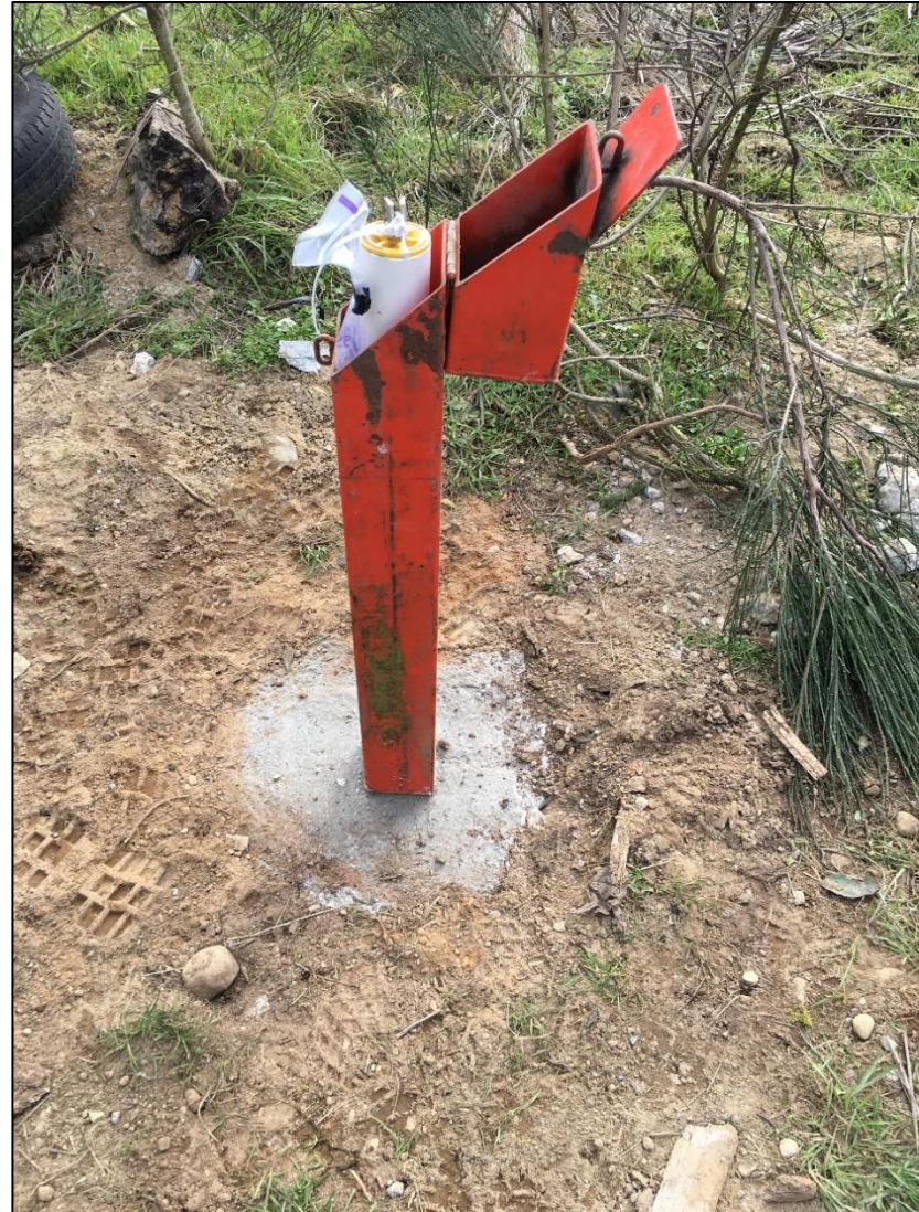
Photograph B6 (RIGHT): Looking down and south at MW12-3 after the well was repaired and the surface seal replaced.
