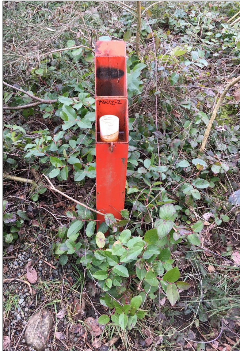
Photograph B2 (RIGHT): Looking down and northeast at MW12-2.
