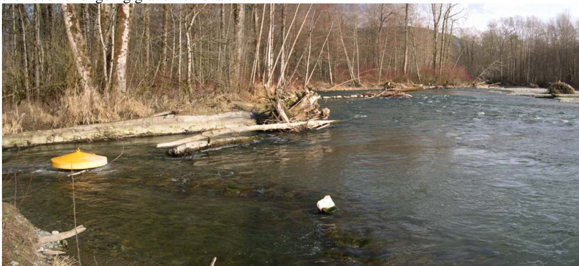
Photo 8.4: Downstream view of lower Fish Gut Alley side-channel intake showing avulsing mainstem flow and proposed installation of ballasted LWD intake feature.
