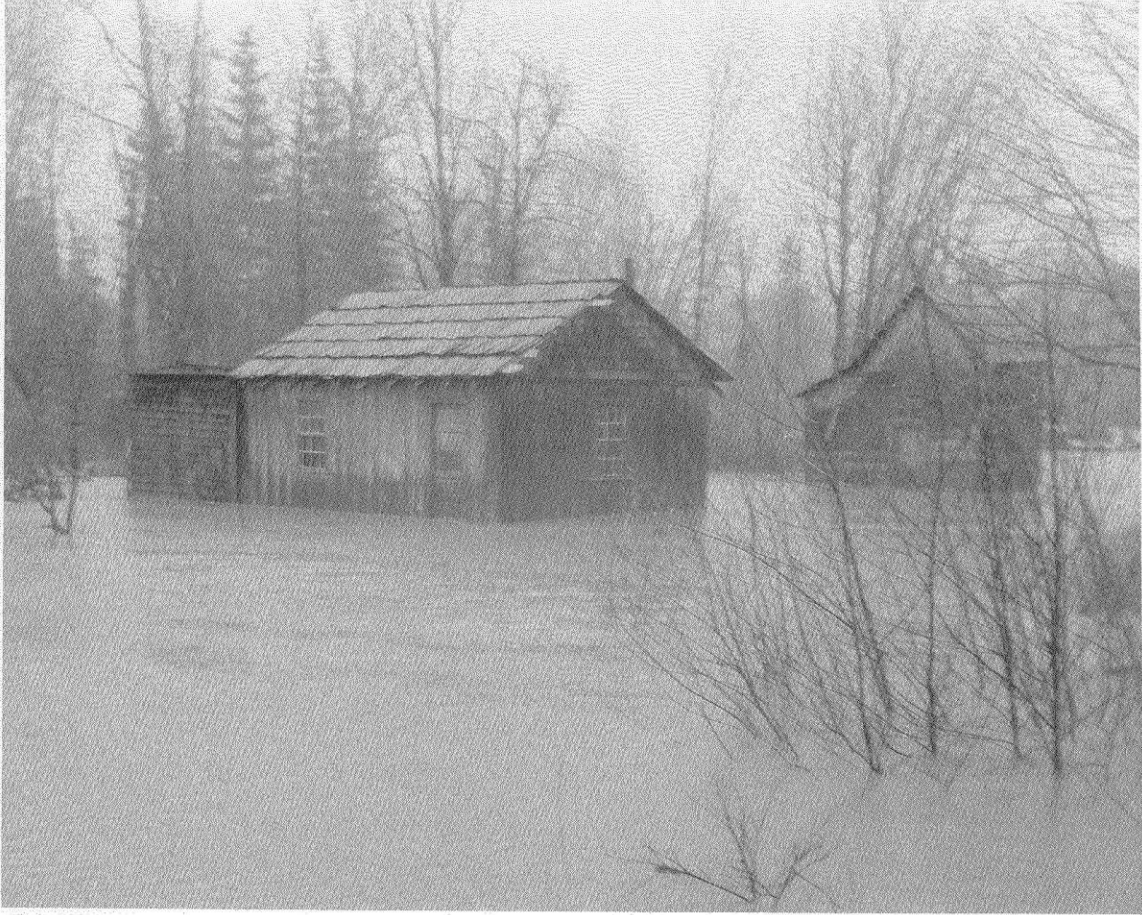
Flooding from Koksilah River on Cowichan Tribes land.
