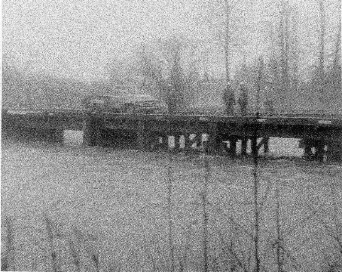
Log jam starting to form at upstream side of bridge.
