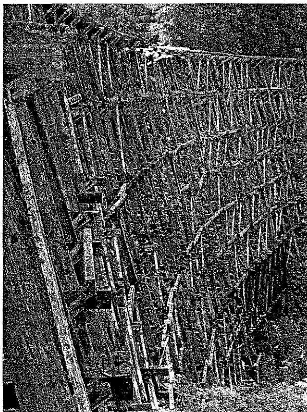
Kinsol Trestle prior to rehabilitation work beginning
