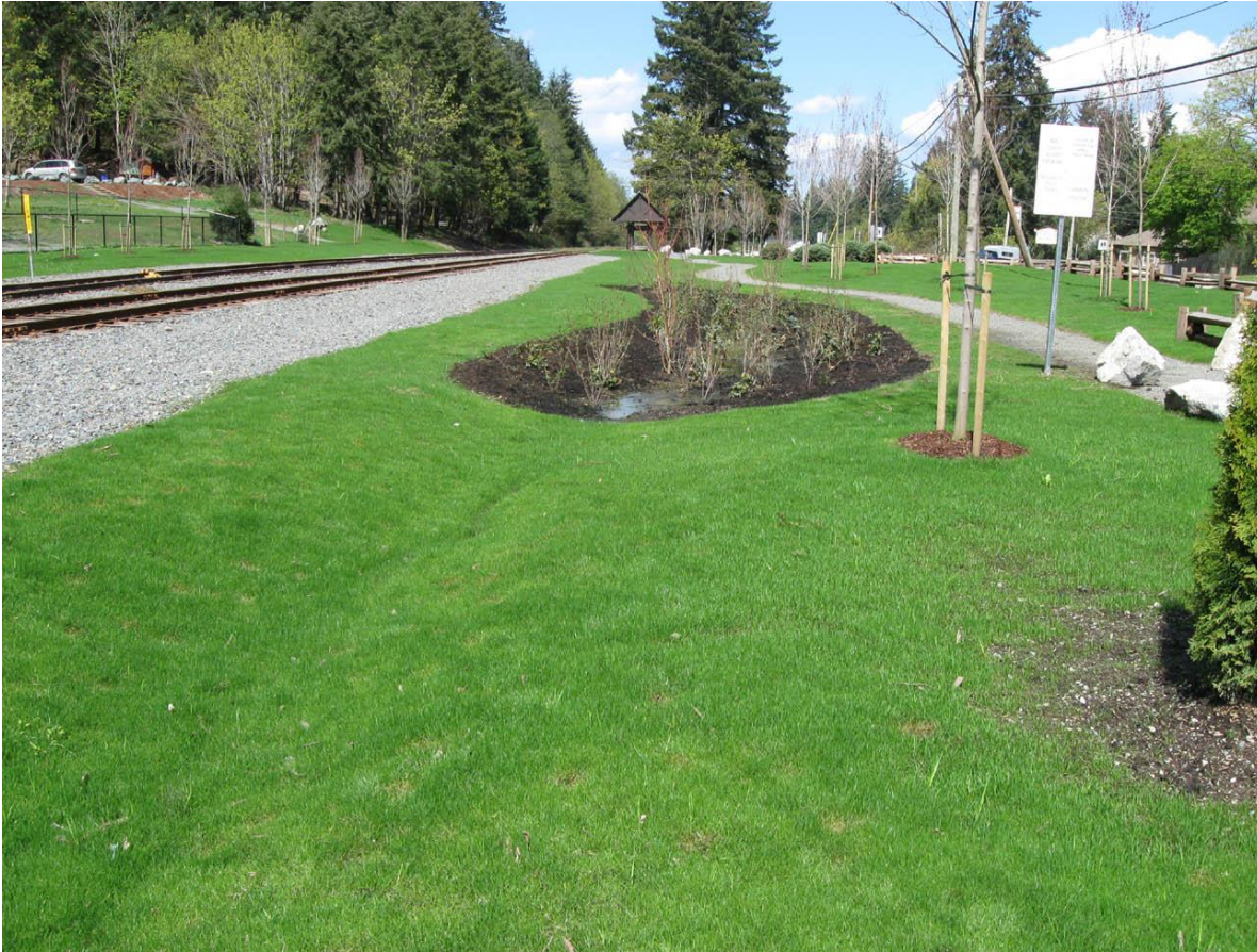
Cobble Hill Train Station - Storm water infiltration swales contribute to storm water management in a way that improves the local ecosystem and offers a new visual aesthetic.
