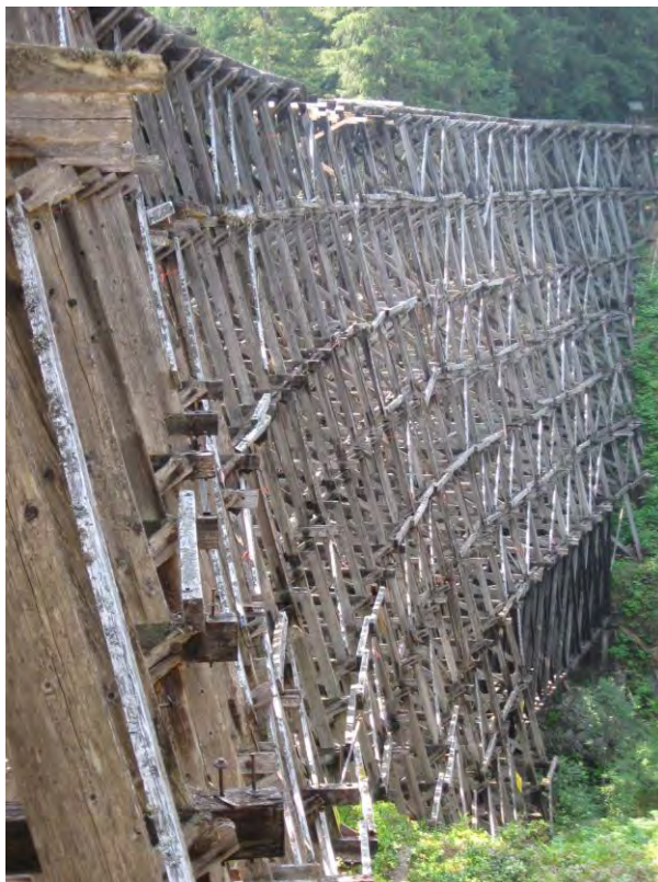
Kinsol Trestle prior to rehabilitation work beginning
