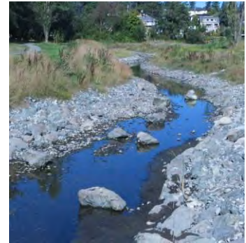
Stormwater infiltration swale
