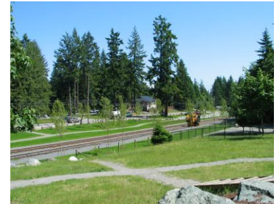
Train Station area upgrade adjacent to the E&N Railway, formerly a gravel parking area.
